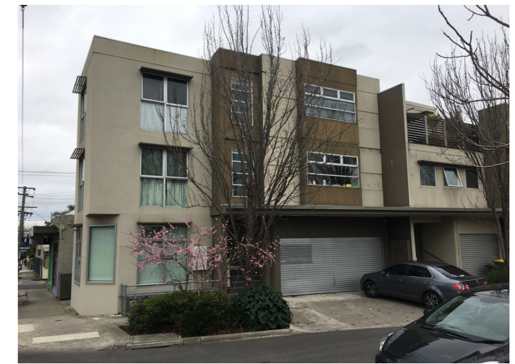
TOWNHOUSES ON WEST SID OF RAILWAY LINE ALONG SCOTT STREET
