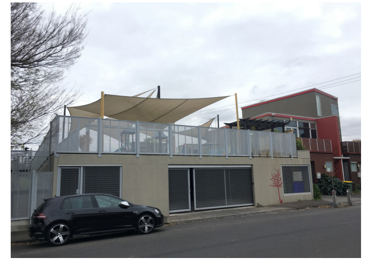
EXISTING TWO STOREY SECTION AT NORTHERN END ALONG HERBERT STREET
