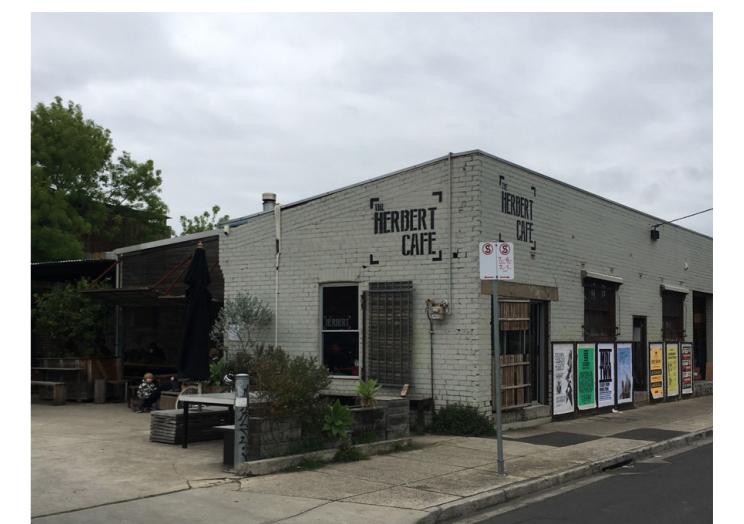
COMMERCIAL BUILDING ON CORNER OF ARTHURTON ROAD AND HERBERT STREET.
