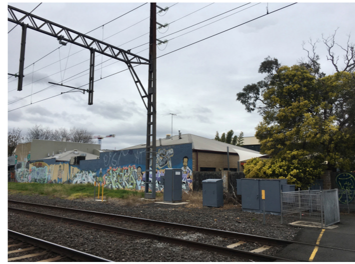
SUBJECT SITE FROM RAILWAY LINE ON SOUTH WEST CORNER.
